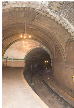
A subway tunnel entering the abandoned City Hall Station, New York, June 2018.
