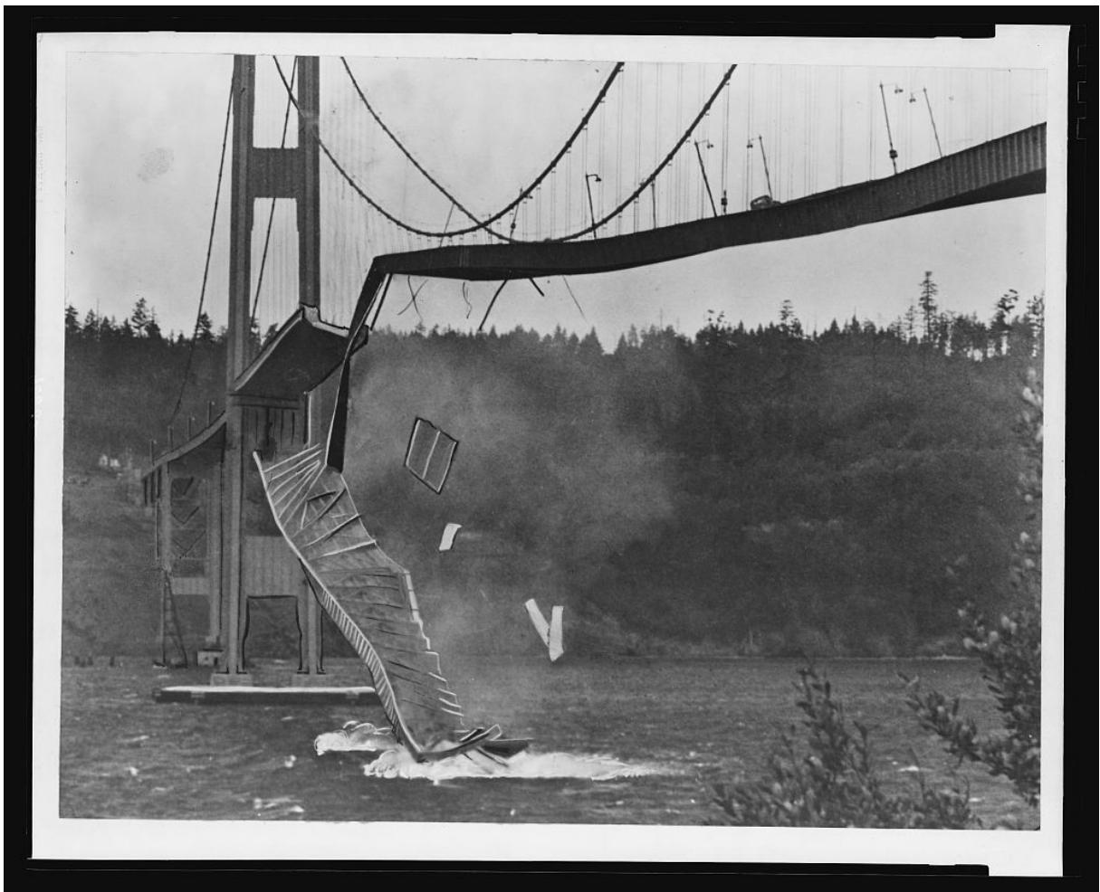
The collapse of the Tacoma Narrows Bridge, 1940. Library of Congress photo archive.
