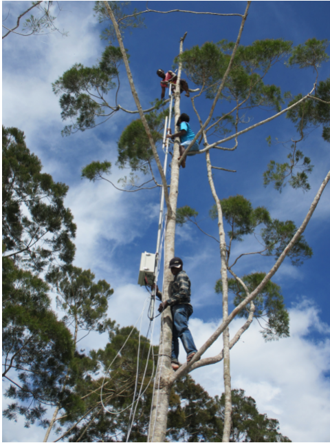
Figure 7: Installing the Village Base Station in rural Papua, Indonesia.
