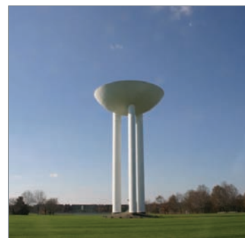
The Bell Labs water tower.
