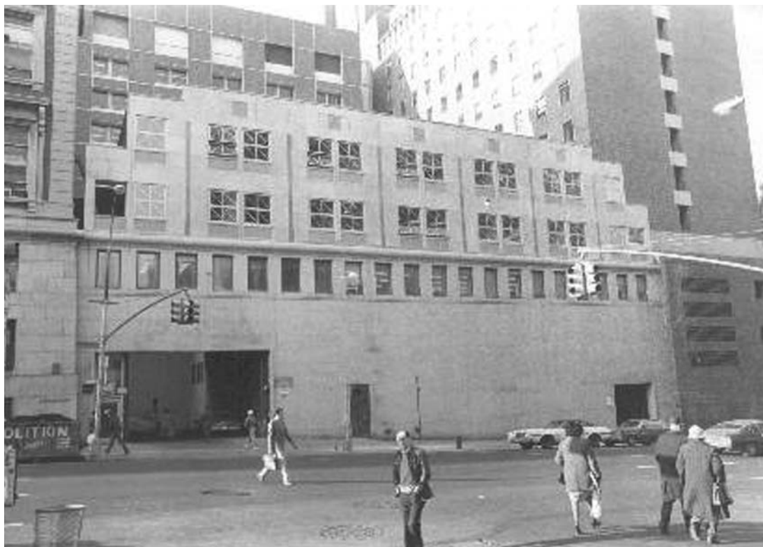
CS Building exterior construction completed, December 1982.
