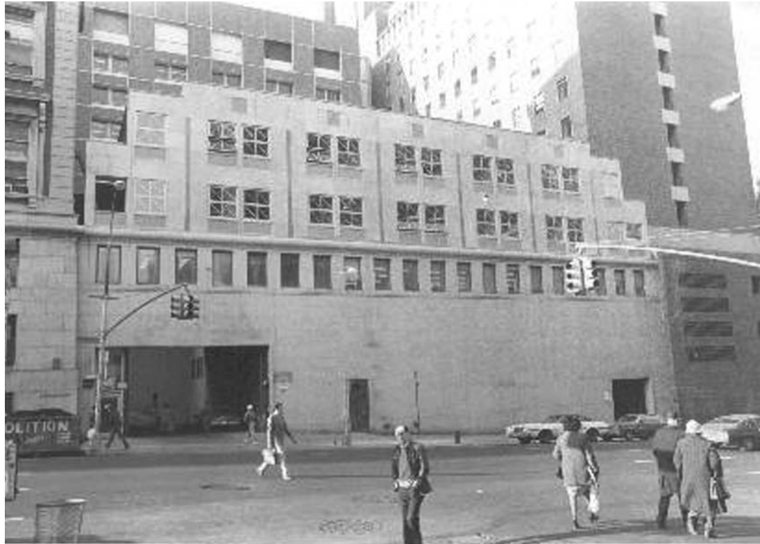
CS Building exterior construction completed, December 1982.
