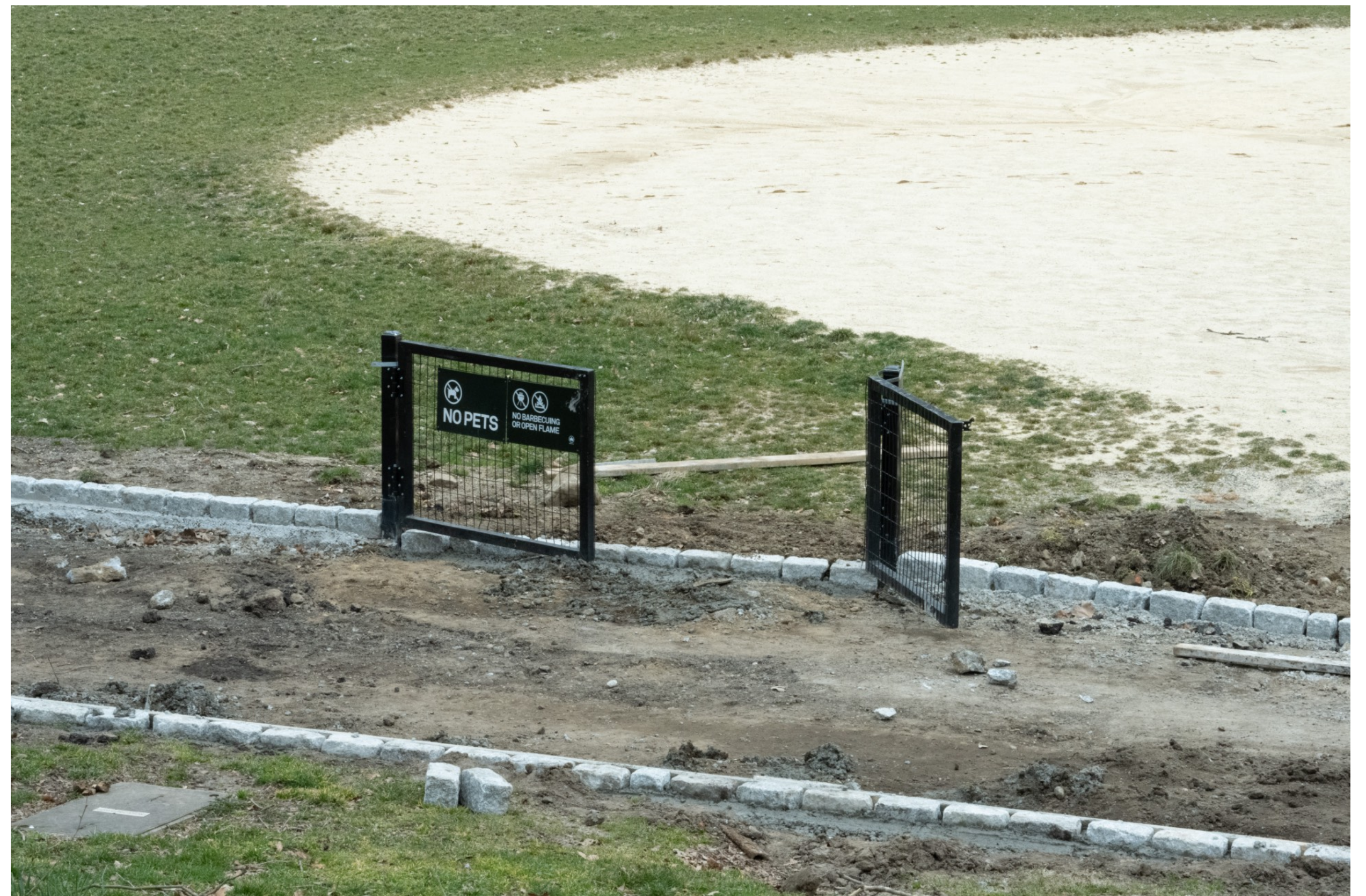
Morningside Park, March 2023
