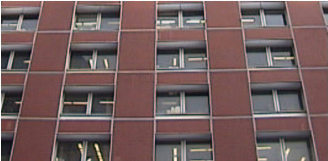
Figure 7.1: A building facade exhibiting repetitive feature patterns
