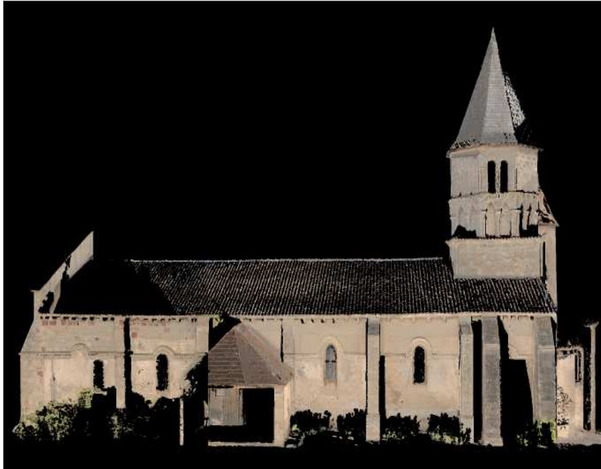
Fig. 13 Albedo map for the south facade of Saint Marie, Chappes, France.
